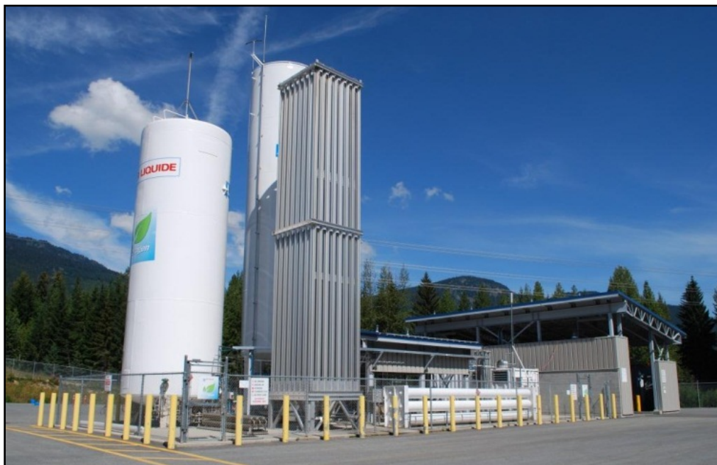
Figure 5. Air Liquide hydrogen station at Whistler Transit Centre
