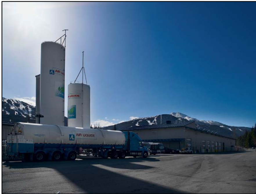
Figure 6. A delivery tanker fills the Whistler Transit station with liquid hydrogen. Photo courtesy of Air Liquide
