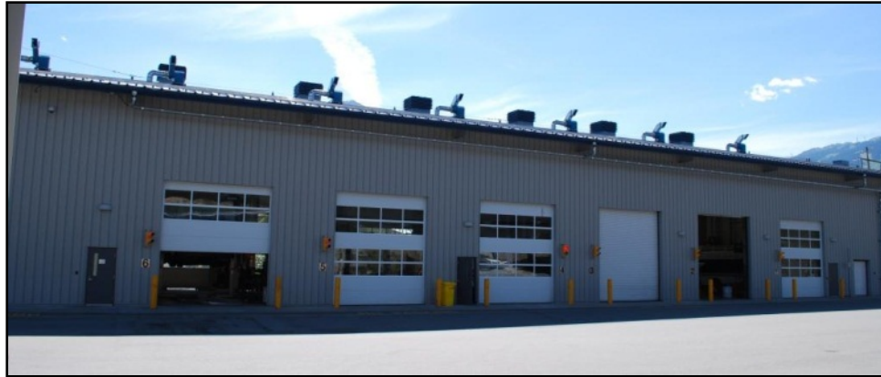
Figure 9. Whistler Transit maintenance facility
