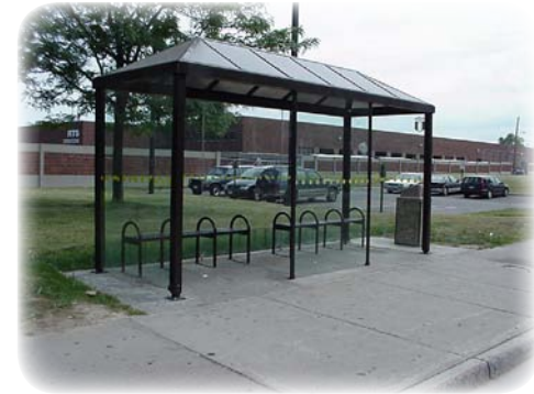
This shelter in Rochester, New York, provides two openings for entering and exiting, as well as wind protection from the northern climate.
