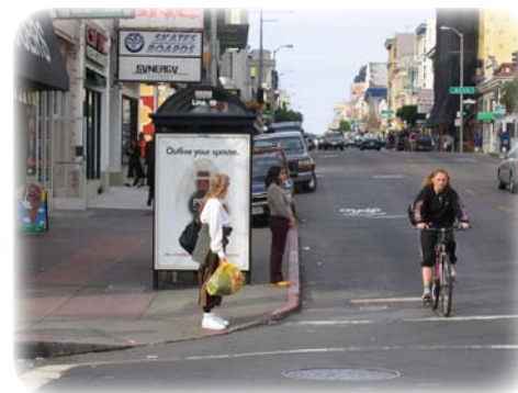
A bus bulb in San Francisco, California. The bus stop area is extended into the parking lane and incorporates a shelter that does not impede the pedestrian right of way. The bulb allows the bus driver to pull up flush to the curb to facilitate the boarding and alighting of passengers.
