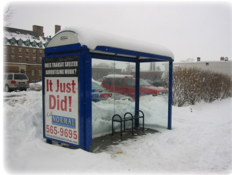
This bus stop in Buffalo, New York is not accessible, lacking a plowed path to the shelter. Bus patrons with and without disabilities will have difficulty getting to the stop and getting onboard the bus due to the thick layer of snow.
