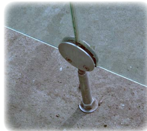
The glass panels of this bus shelter are raised above the ground to accommodate cleaning, but not so high as to create a problem for white cane users. Picture taken in Toronto, Canada.
