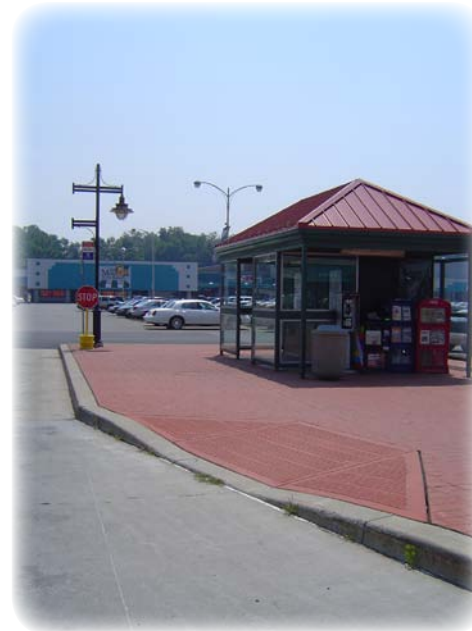
Example of a curb ramp leading to a bus stop in Buffalo, New York.
