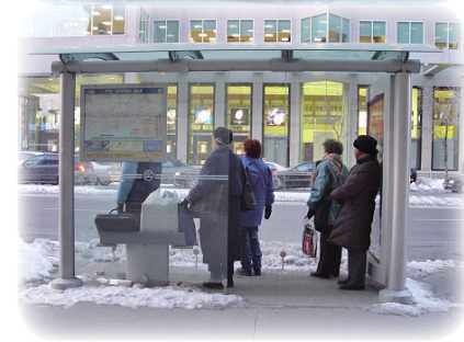
These two shelters in Toronto, Canada, open onto the sidewalk to provide protection from snow or water splashed by moving cars. The shelter is enclosed except for the entranceway to protect against inclement weather.
