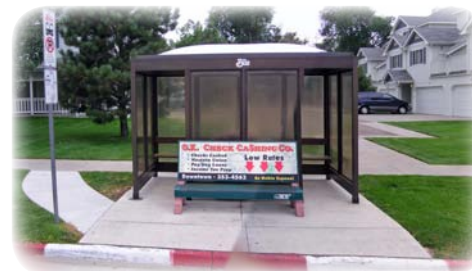
The exterior bench at a stop in Greeley, Colorado is poorly placed, obstructing accessibility on the landing pad and into the shelter. The stop would otherwise be accessible, with a path connecting the stop to the sidewalk and a suitable landing pad, if the bench was not placed in its current location.
