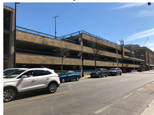
Figure 6 State Street Campus Garage
