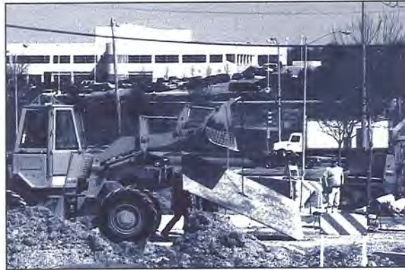
Construction begins on the West Transfer Point.
